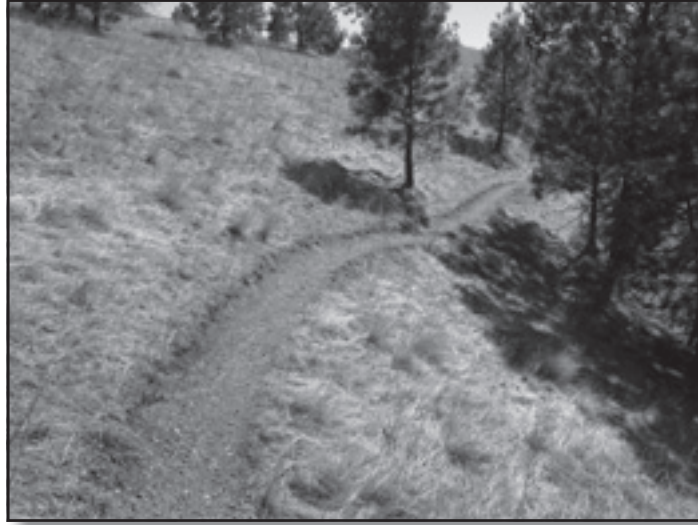
Figure 1—A rolling contour trail resists erosion.
