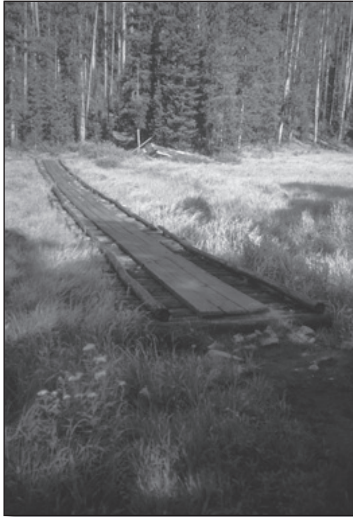
Figure 48—Standard puncheon is slightly elevated above the ground.
