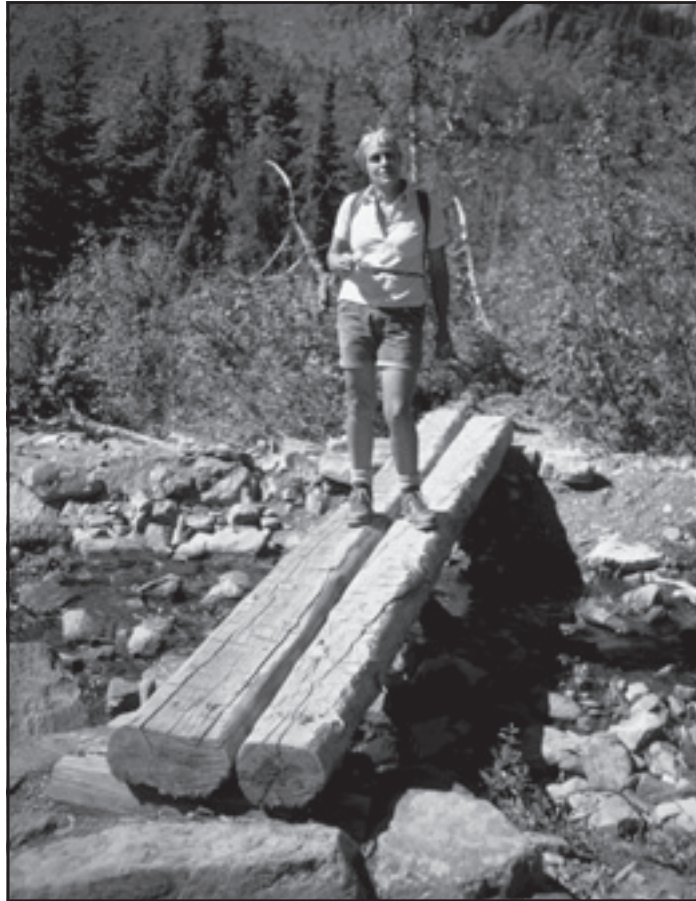
Figure 63—A log footbridge. The sill can be notched to accommodate the logs, but not vice versa. Photo has been digitally altered.
