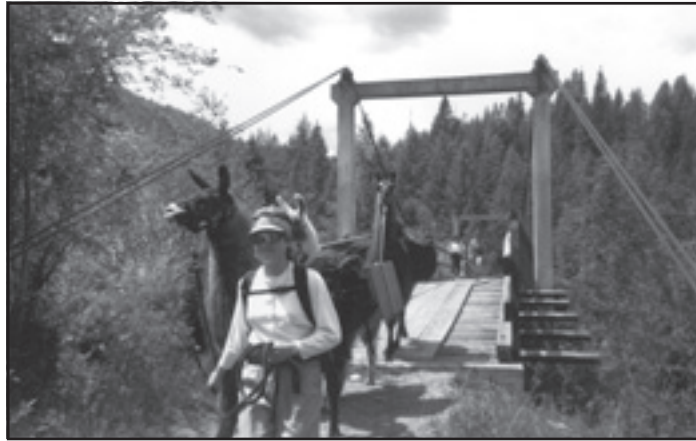
Figure 64—A suspension trail bridge typical of the Northern Rockies.
