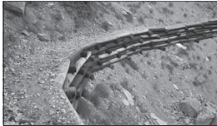
Figure 76—Crib walls help keep compacted fill in place.
