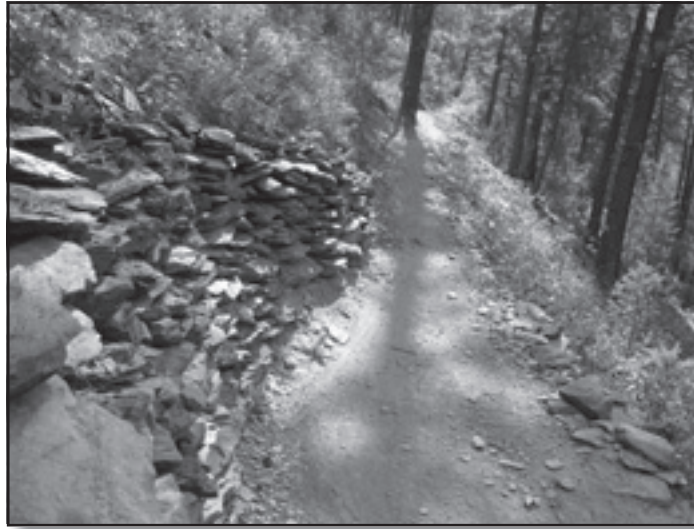
Figure 74—A rock retaining wall holding a steep, excavated backslope in place.
