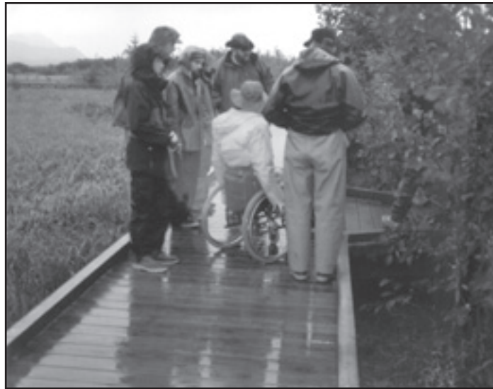
Figure 34—This boardwalk relies on pilings for support. Helical earth anchors also could be used to support the structure.
