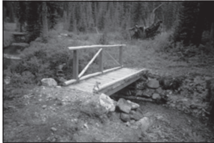
Figure 62—A simple footbridge with a handrail.
