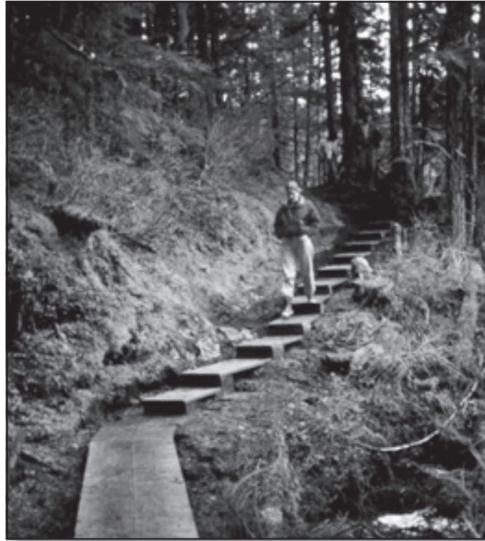
Figure 79—A step-and-run boardwalk in Alaska.
