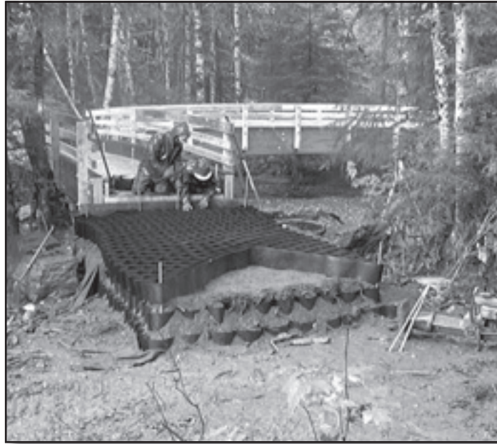
Figure 38—Geocells are good for tread reinforcement and help hold fill in place.
