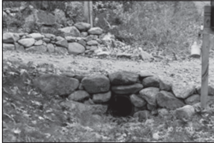
Figure 59—Culverts are a good option for moving small volumes of water under a trail.
