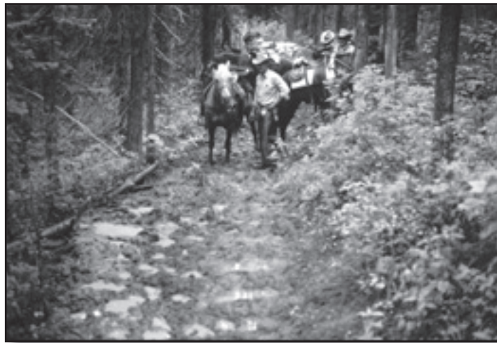
Figure 9—Standing water results in soft, boggy tread.
