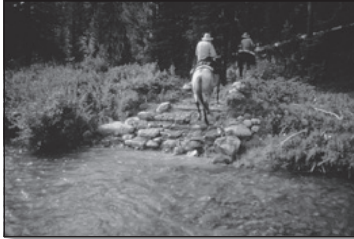
Figure 57—Fords should be established in wider, shallower portions of a stream. Approaches should climb a short distance above the high-water line.
