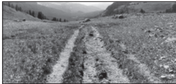
Figure 89—A candidate trail for a turnpike or rerouting, followed by reclamation of the old trail.
