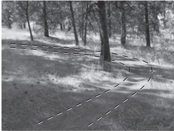
Figure 67—Climbing turns are easier for packstock and cyclists to negotiate than switchbacks.
